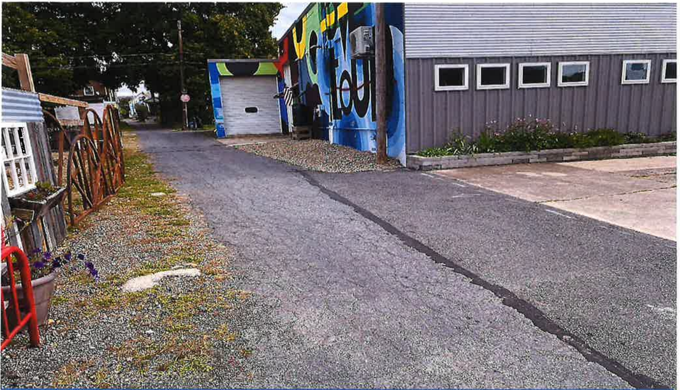
SIDE VIEW FROM HORNER STREET
