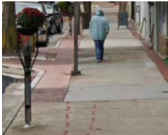
Sidewalks are uneven and obstructed light-posts and other street furniture
